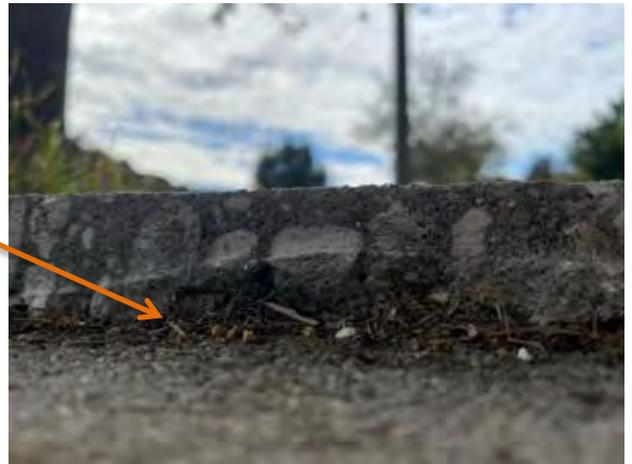
Example of a  $1\frac{1}{4}$ -inch high “Most Severe” hazard located on Eve Court.
