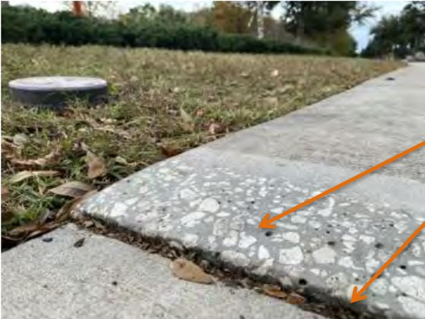
Example of a hazard on Promenade Parkway where a poor repair attempt was made with a grinder, leaving a  $\frac{3}{8}$ -inch hazard on the edge of the panel and damaging the aggregate of the panel. Hazards like this must be repaired properly by PSSC to remove the remaining portion and provide a proper slope. These types of hazards are **included** in this proposal.
