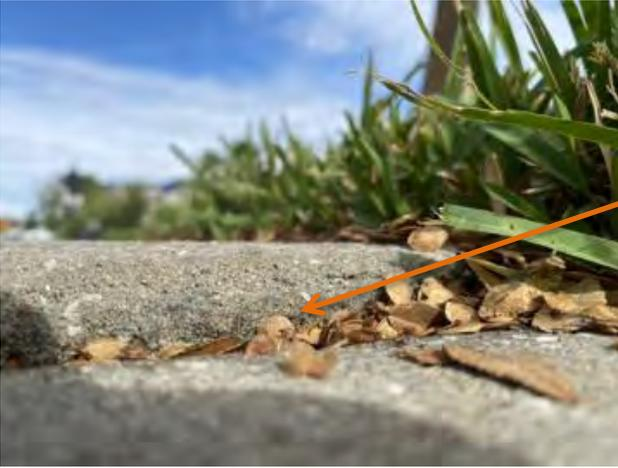
Example of a  $\frac{3}{4}$ -inch high “Severe” hazard on Trails Edge Boulevard.
