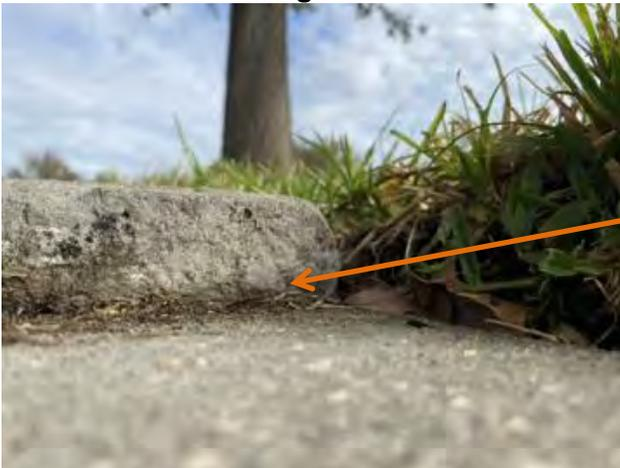
Example of a  $1\frac{1}{2}$ -inch high “Most Severe” hazard located on Eve Court.
